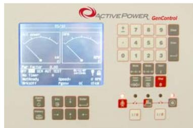
FIGURE 15: EXAMPLE OF A DIGITAL ENGINE CONTROLLER
